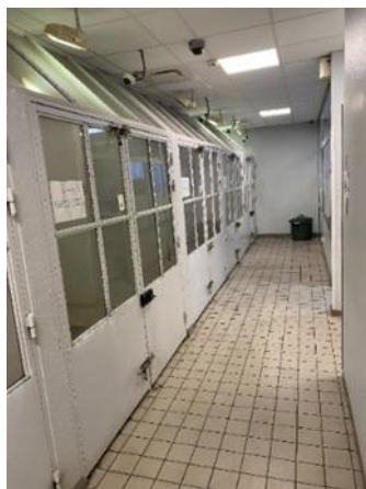
Couloir cellules GAV
