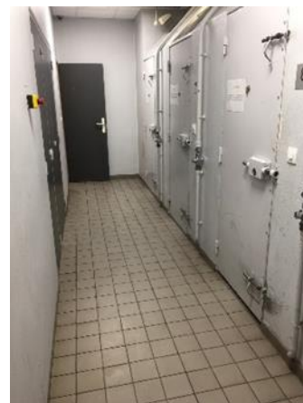
Couloir cellules IPM
